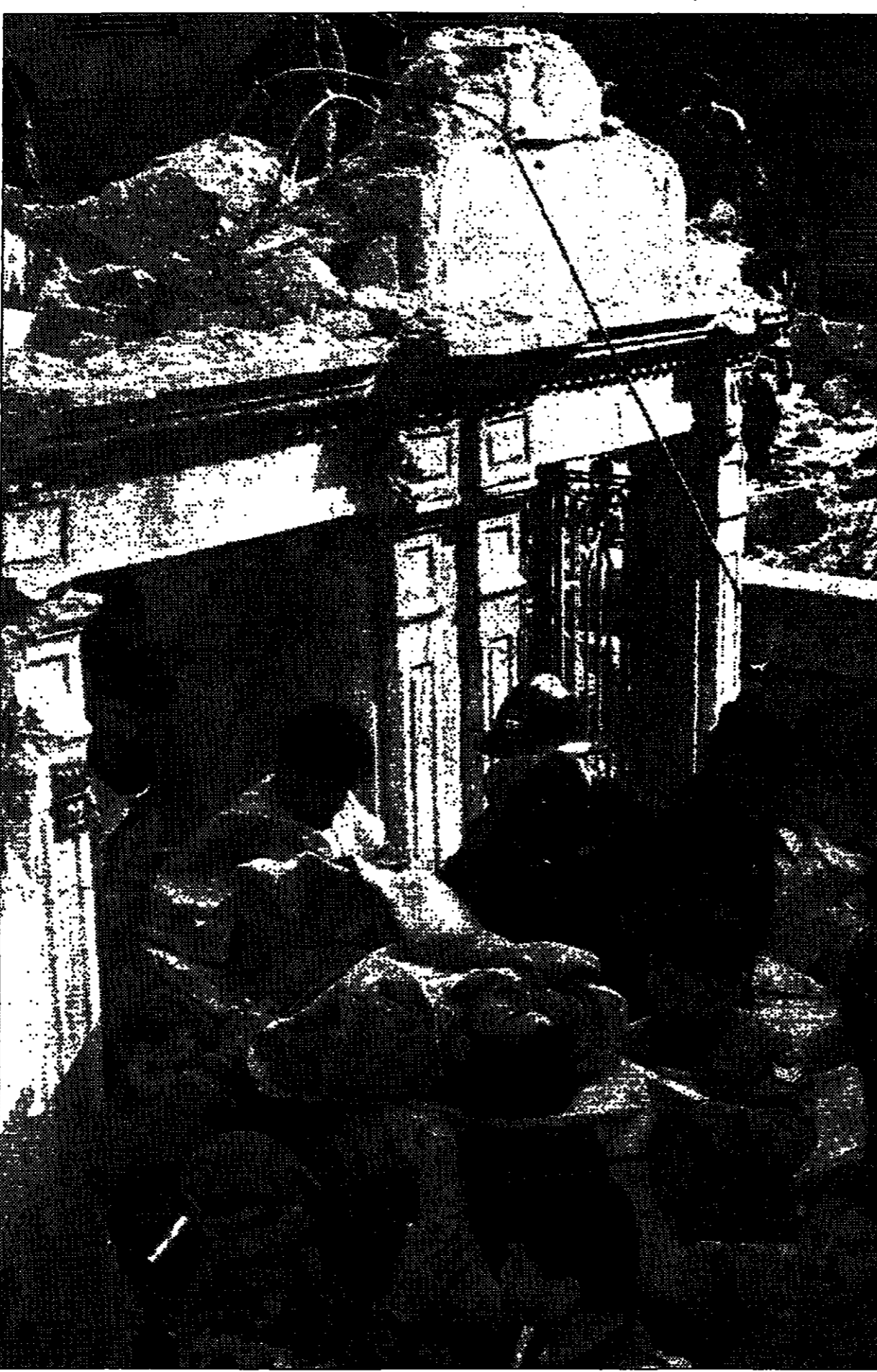
Reconstruction effort... Rescuers carry out a man injured when a building in central Beirut collapsed yesterday after workers started to destroy its foundations to drive out squatters. At least two died, eight were hurt and up to 15 were believed to be buried in rubble. The government-sponsored Solidere firm is rebuilding the area. PHOTOGRAPH: ALI MOHAMMED
